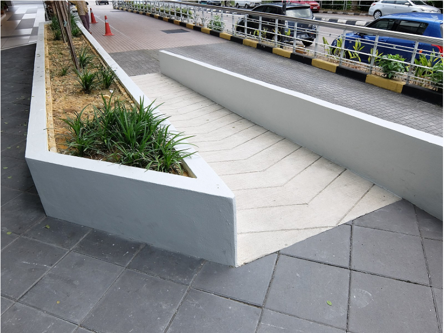
Pelangi Tower - Wheelchair Ramp from Chongjian licenced under CC.BY-SA.4.0
